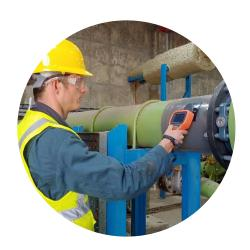
Thickness readings could be taken free of human error using WAND
