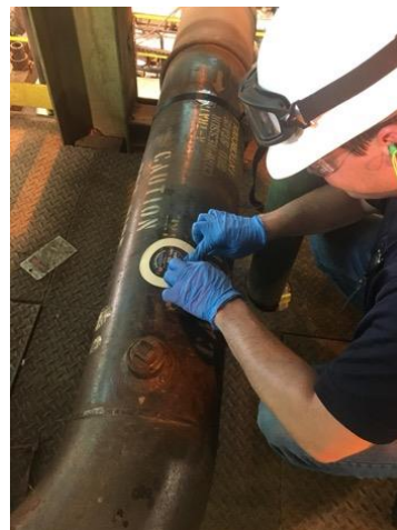
Examples of sensors installed on the tank head and connected pipework
