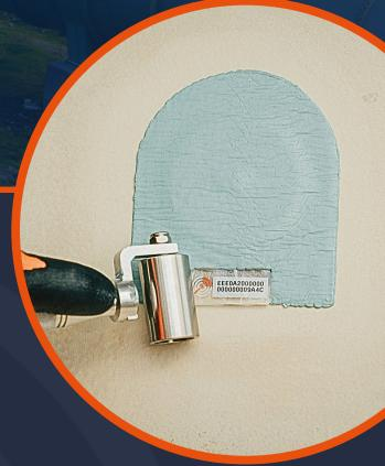
WAND Sensor Installation at Unpiggable Locations Along Natural Gas Pipelines
