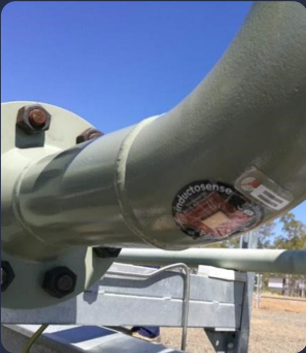
WAND sensors installed at sand erosion examination points (prior to coating)
