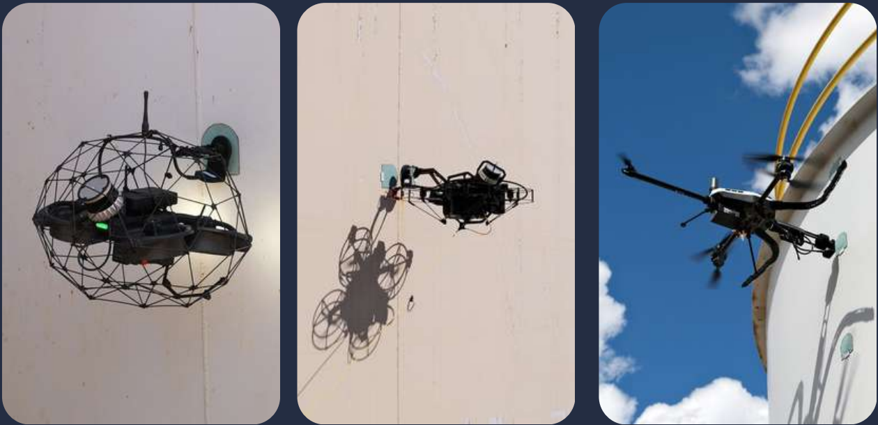
Figure 1: Sensor locations and drone-enabled data collection from tank assets
