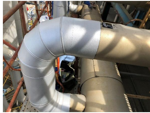
Measurement locations underneath insulation, accessed using the ECHO45
