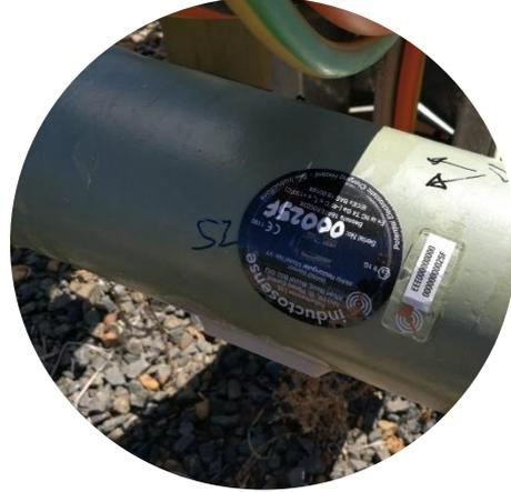
WAND sensors installed at sand erosion examination points (prior to coating)
